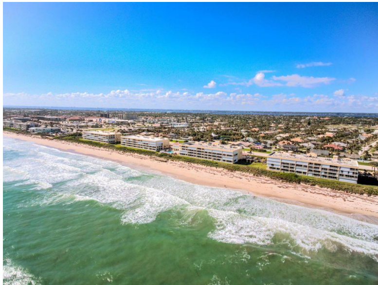
Figure 1: View of Parcel and Structure
