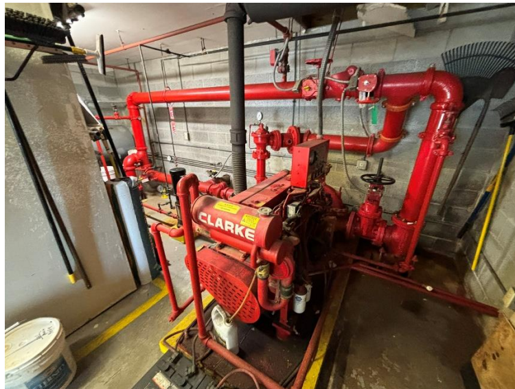
Figure 4: Fire Pump
