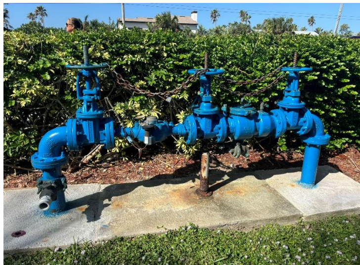
Figure 6: Backflow Preventer
