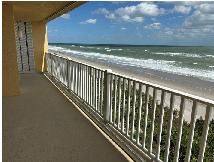
Figure 11: Typical Guardrails on Balconies
