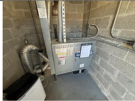
Figure 8: Elevator Room, No Visible Cracks
