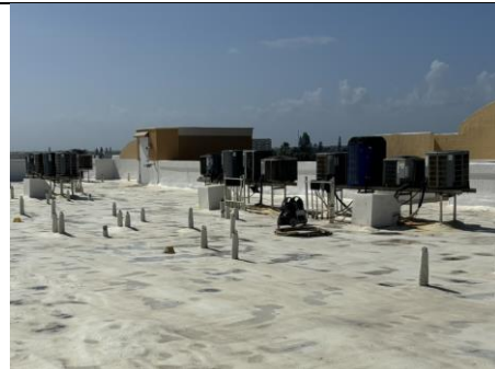
Figure 14: Flat Roof in Good Condition
