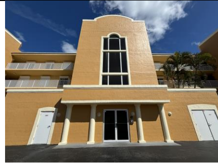
Figure 6: Building in Good Condition
