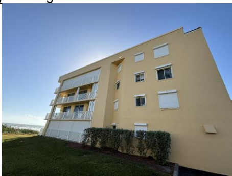
Figure 9: Mansory Walls in Good Condition
