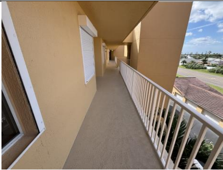
Figure 7: Typical Walkway, No Visible Cracks
