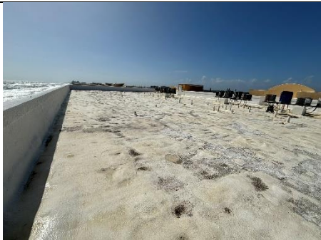
Figure 13: Flat Roof in Good Condition
