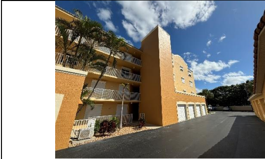
Figure 5: Building in Good Condition
