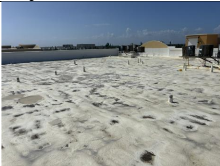
Figure 17: Silicone Rubber Coating Roof System in Good Condition
