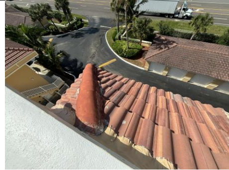
Figure 16: Clay Tile Roof in Good Condition
