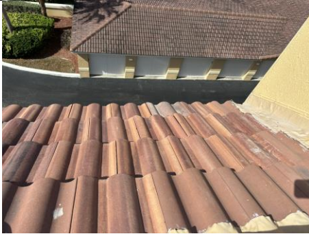
Figure 15: Clay Tile Roof in Good Condition
