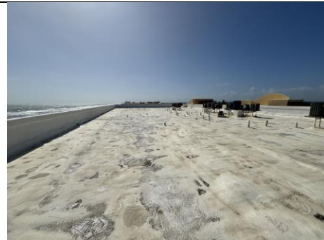
Figure 18: Silicone Rubber Coating Roof System in Good Condition
