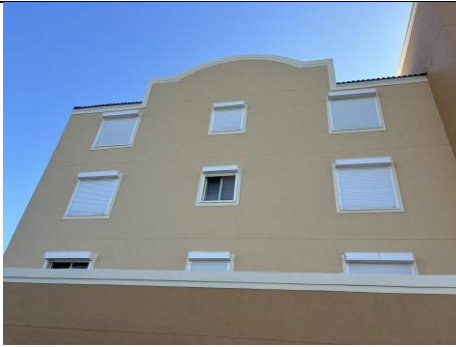
Figure 11: Stucco Finishes in Good Condition
