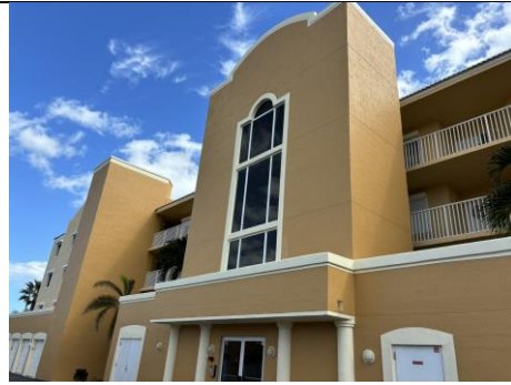
Figure 12: Stucco Finishes in Good Condition
